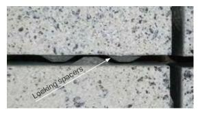
SCADA is coming with an efficient locking spacer system. This technology enables pavement to remain stable even when it is subject to strong dynamic loads, such as those generated by sudden braking of vehicles going downhill. The locking spacers are coming by size of 40 mm (VZ4) and 50 mm (VZ5), fitted on the sides of the slabs and are invisible once placed. It is not possible to combine VZ4 and VZ5.
