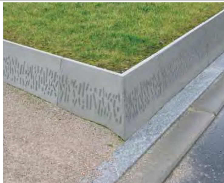
Dunkerque (FR) retaining walls with structure
